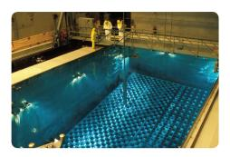
This "high-level" nuclear waste is initially stored in a stainless steel-lined water pool in the Callaway Plant's Fuel Building, located adjacent to the Reactor Building. The plant has sufficient storage space in the spent fuel pool until the year 2020, and Callaway planners are considering the construction of dry cask storage to provide additional space—as many plants have already done.
