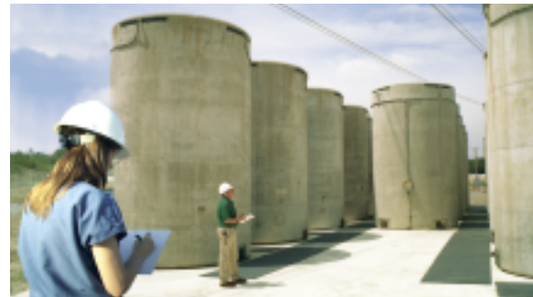
Nuclear energy facilities store used fuel safely and securely on site in steel and concrete containers.
