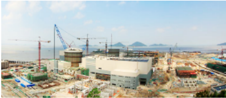
More than 65 nuclear energy facilities are under construction around the world, including this Westinghouse AP1000 in China.
