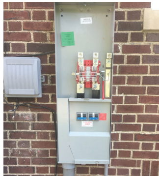
400 Amp With Breaker Safety Lever By-Pass
