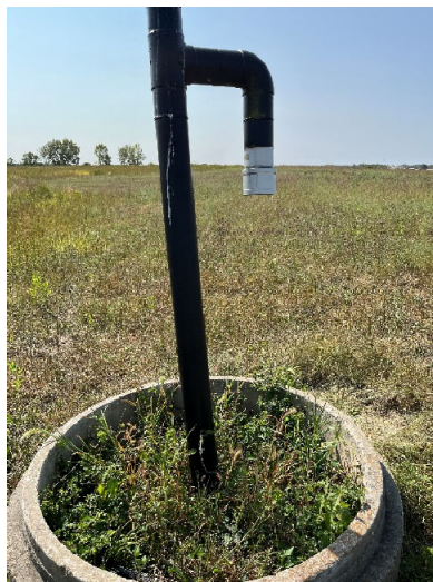
Vegetation Observed in Vent Pipe Cement Barrier
