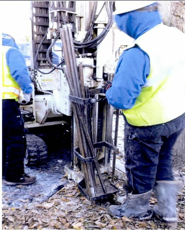
Photo 7: 304-E-3-Boring Installation
