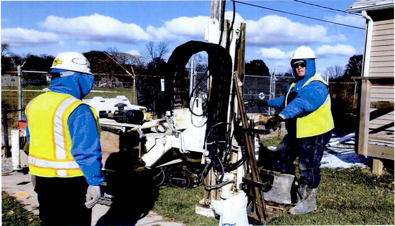
Photo 1: 304-W-1 Boring Installation Using Geoprobe 6610DT
