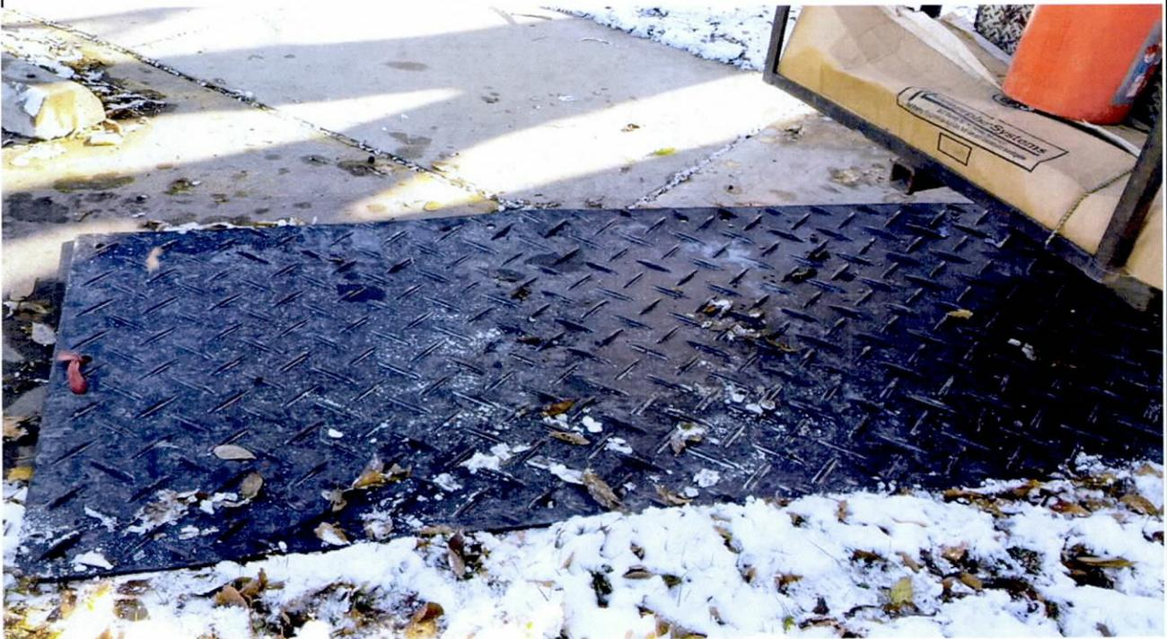
Photo 6: Mud Mats used at 304-E-3 to avoid damage to grass and pavement
