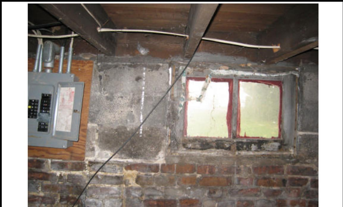
**PHOTO 15:** View of window along south wall of basement. There are several gaps between window frame and bricks & cinder blocks in this area and throughout basement.
