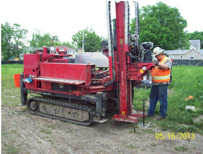
Above: DPT installation of injection locations – two screen depths per location.
