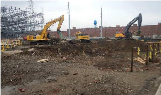
The project work involves excavation of an expected 27,280 tons of material from the Tower Area and an expected 147,060 tons of material from the Phase 3 Area. Considering these depths typically are 20 feet or greater from the existing ground surface, excavation will require the installation of perimeter excavation support systems that will be installed by Goettle.
