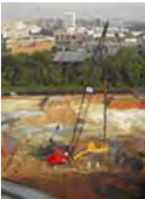
Ex-situ treatment included conditioning of tar and tar-like materials with other soils and quicklime. Approximately 5,000 tons of heavily impacted soils were treated, stockpiled, tested, and transported off-site using 175 tons of quicklime. In-situ stabilization was performed with a 12-foot-diameter mixing/injection tool powered by a high-torque drill transmission attached to a 150-ton crawler crane.
