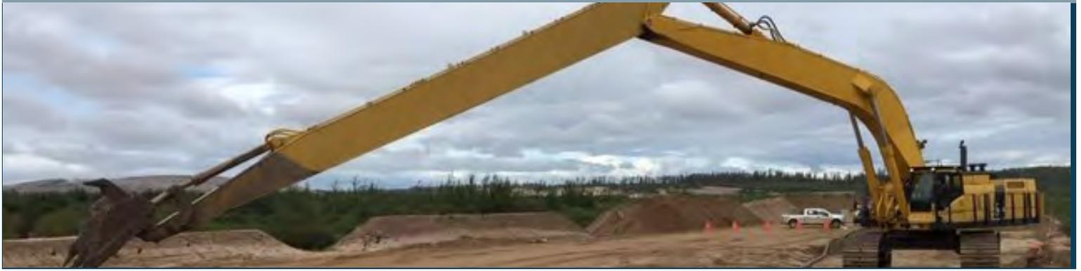
slurry is designed to be in the fluid range during the excavation process. The slurry stays in the trench and is allowed to set. Typical CB slurry will attain a butter-like consistency overnight and a clay-like consistency after fully hardening (generally 28 to 56 days).
