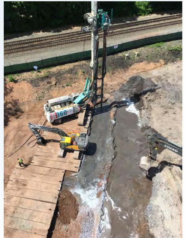
Large diameter mixing can also be used to install geotechnical elements. The term deep soil mixing (DSM) often refers to the use of multi-auger soil mixing rigs that are most commonly used to install linear elements, such as cutoff walls or shear panels. DSM auger configurations are specific to each contractor, but typically include 3 or 4 relatively small (3' to 4') diameter augers spaced evenly apart.
