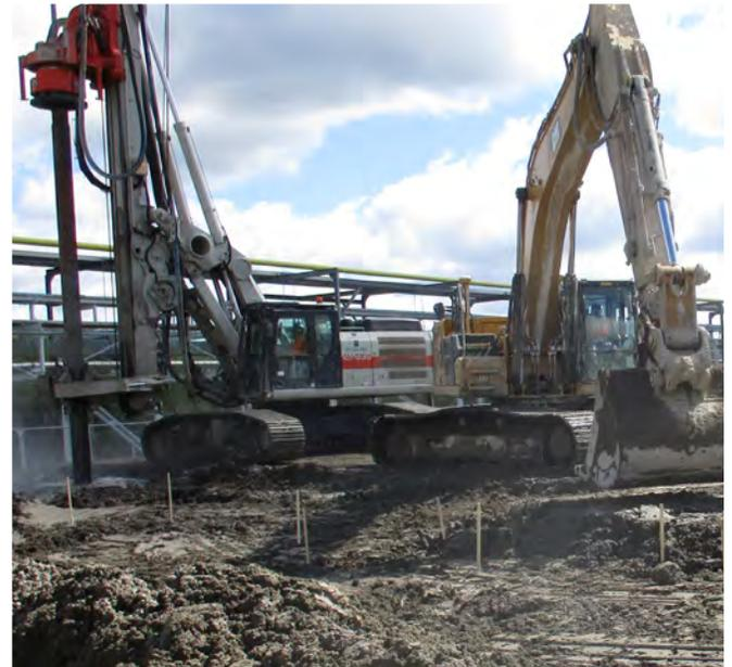
Logistical challenges included site access constraints including height restrictions and site access bridge weight restrictions for equipment, ISS around pile cap locations to maximize the amount of impacted soil remediated via ISS, ISS nearby overhead utilities including pipe racks, and sequencing of ISS to support drill rig stability during mixing.
