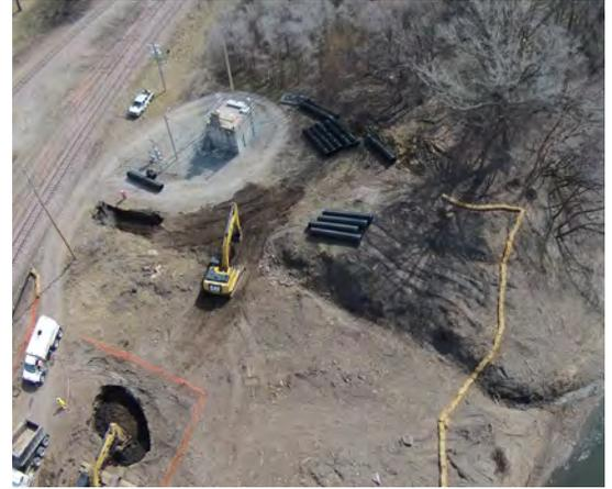
ENTACT installed temporary dams to divert water flow around the work area, along with a retaining wall made of ISS columns along the bank, to enable the excavation and treatment of impacted sediments located on the shoreline.
