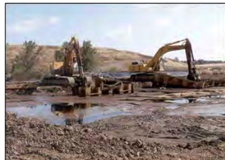
TSCA clay liner and leachate collection system. Construction of a multi-layer RCRA cap. Installation and development of post construction perimeter monitoring well system.
