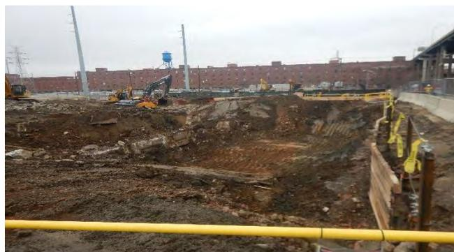
Material will be excavated and loaded into trucks in a controlled to minimize any potential for contamination of the exterior of the trucks. Trucks will exit the site once loaded by travelling across the truck washing area and wheels will be washed to the extent necessary.
