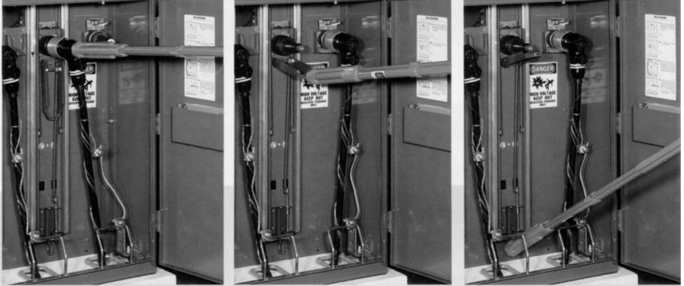
The operator moves the loadbreak elbow to a feedthrough or stand insulator on the parking stand, interrupting any fuse load.
