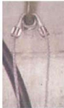
The split grips, used by Ameren to support cables on terminal poles, are as follows:
