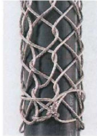
4. Remove the slack from the mesh grip starting at the strand equalizers and working toward the tail end of the grip. Apply one or two cable ties (Stock #40 59 191) to the mesh grip approximately 1 to 2 inches from the tail end of the mesh grip. This may help keep the grip from moving or releasing. The tails of the cable ties should be cut off.
